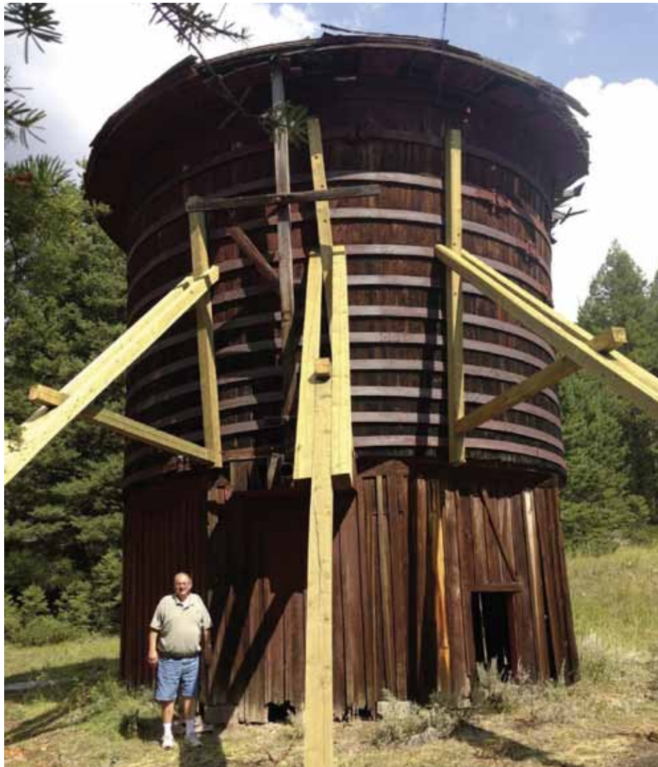
Bill Taylor with the stabilized Elkhorn water tank
