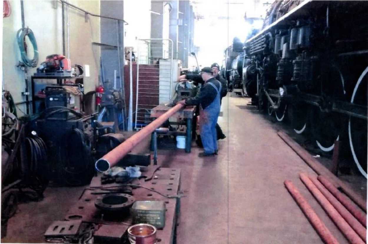
PRPA volunteer members preparing a flue for safe-ending by the contractor
