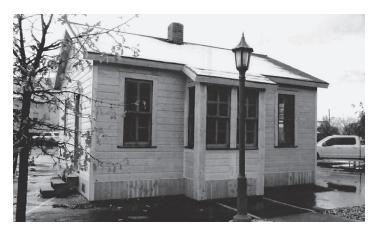
East Helena depot after re-siding with non-conforming materials and practices. Siding and trim will be replaced according to NPS-DOI standards.
