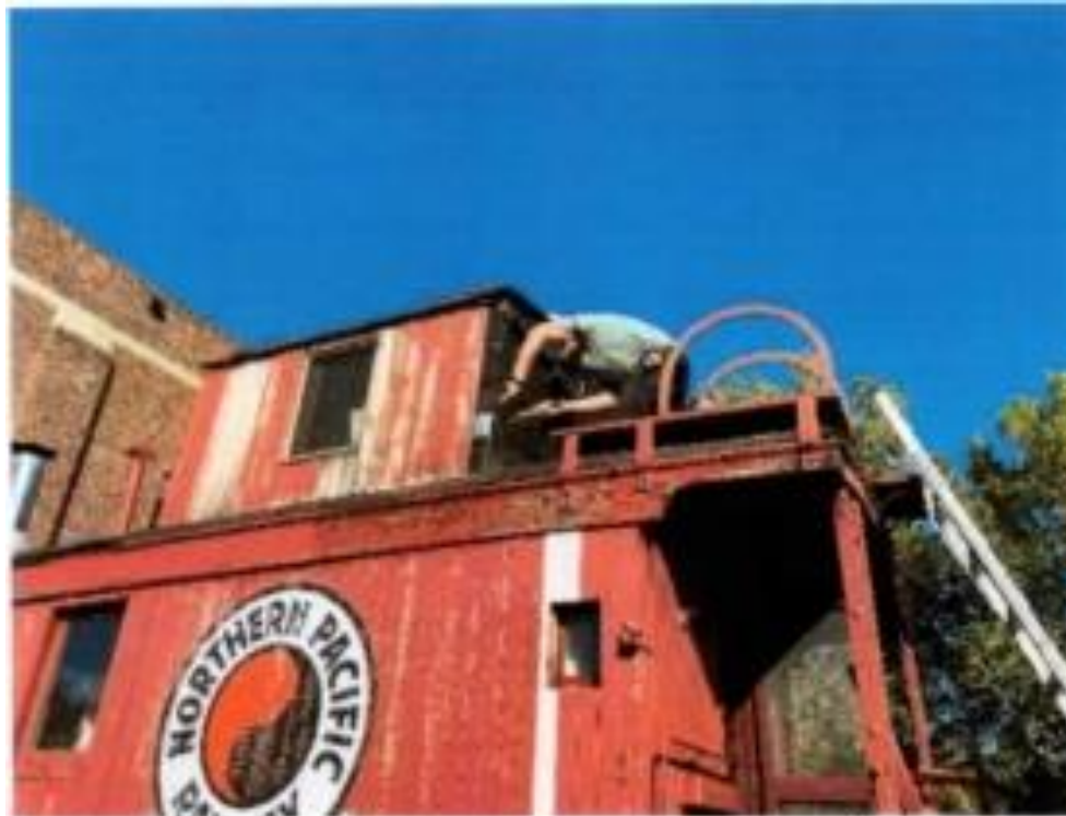
A worker from "The Expert Company" works on the cupola.
